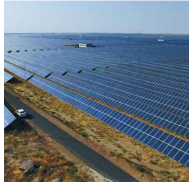
Aditya Birla 650MWp, GJ
